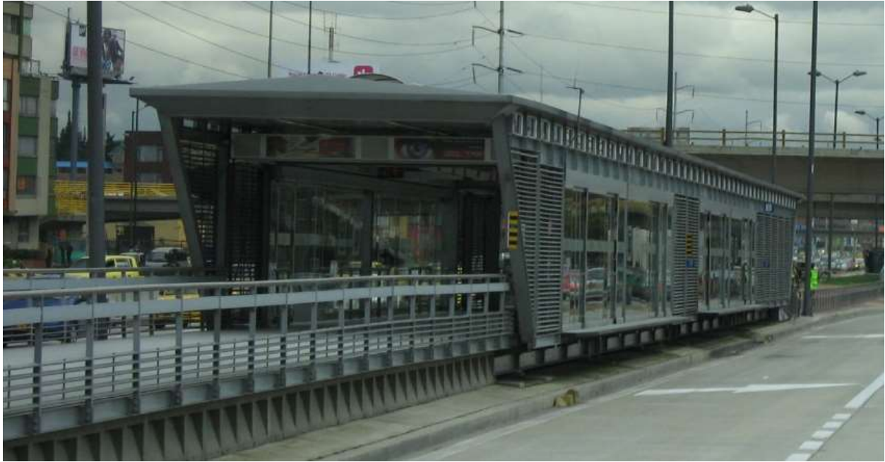
Figure 4.15 Arterial BRT station in Bogotá, Colombia
