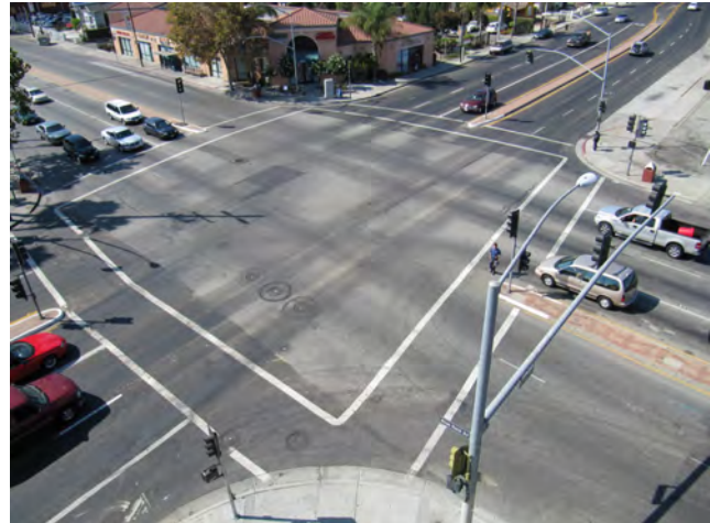
Figure 7: Site of the future King Rd. BRT Station on Alum Rock Ave.
