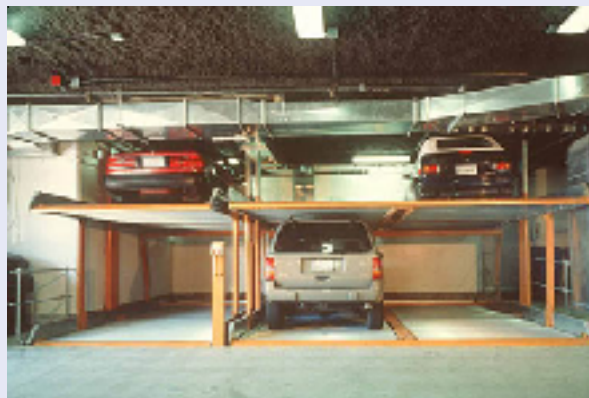
Space-efficient and simple to use, parking lifts like these in the Gaia Building in Berkeley, with independent access to each car, can allow pedestrian oriented ground floor uses.
