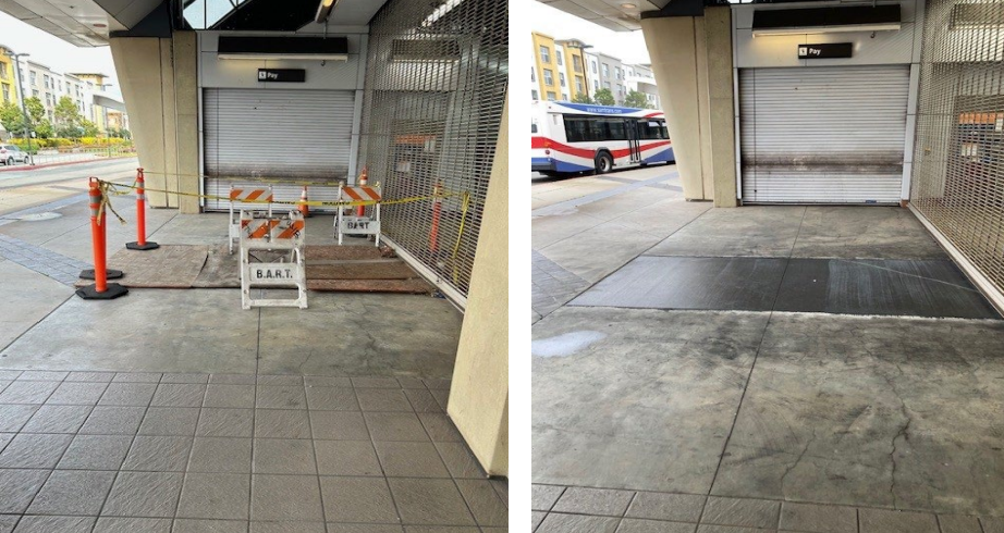
South San Francisco: Repaved Uneven Concrete Pavement
